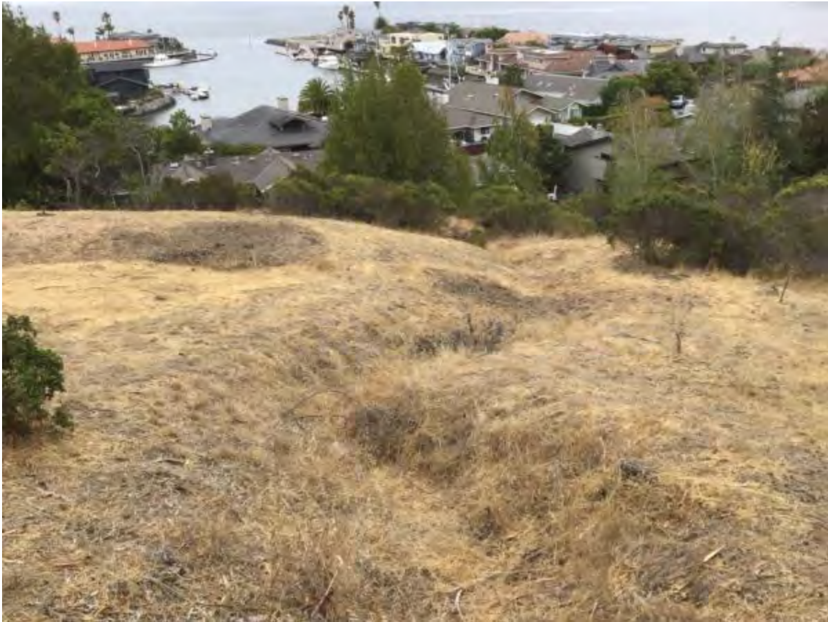
Photo 5. Swale downslope of culvert C1. Note the lack of a well-defined bed, bank, and channel indicating infrequent and low volume flows.
