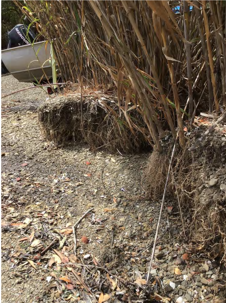
Photo 8. The HTL was delineated in the field using the limits of bank erosion and wrack line.
